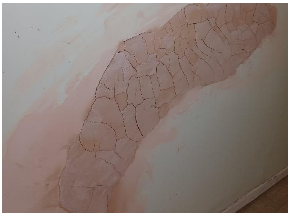
Photo 20: Worst case localised cracking, located on the communal corridor on the 15 th floor level.
