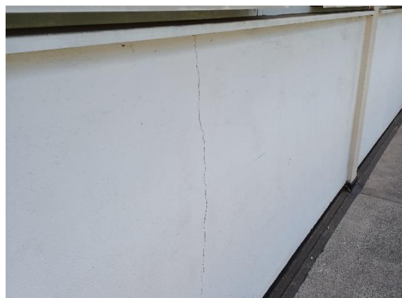
Photo 29: Typical crack severity and location, found in multiple areas within the lobby and the suspended balcony.
