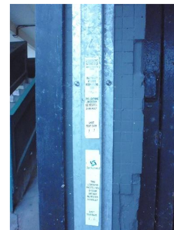
Lightning protection system at main entrance.
