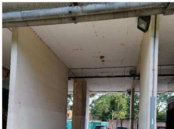
Photo 11: Corrosion staining at soffit level.
