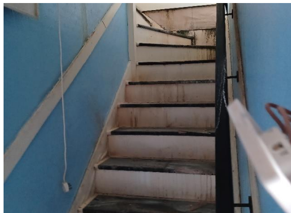
Photo 61: View of staircase exhibiting signs of decay.
