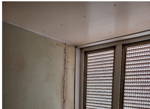
Photo 21: Worst case vertical cracking located at every floor, approximately around the same location.
