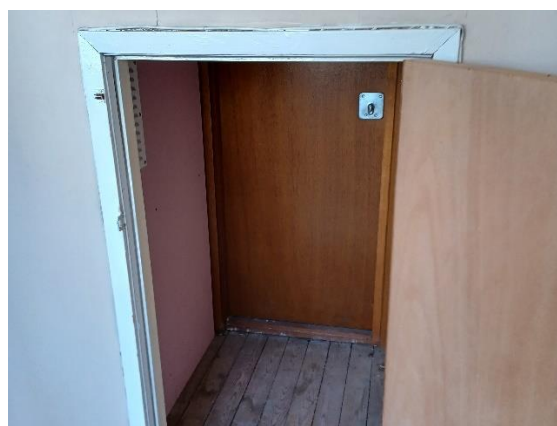
Photo 37: Fire escape hatch, leading to communal corridors.
