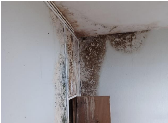
Photo 60: View of excessive ingress affecting bedroom corner and fire escape hatch.
